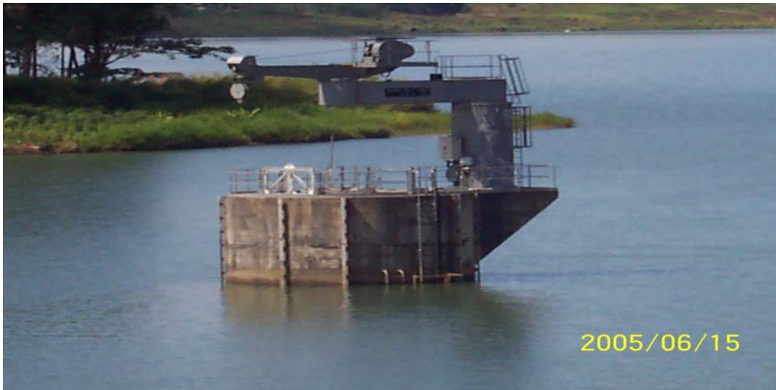
Figure 2: Water Level/Flow Monitoring Station, Yonki, Eastern Highlands Province.
